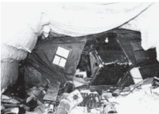
Fig. 6.3 Our sleeping quarters in 1964 – and 5 years later. Already in 1964, it was difficult to pass the hutments due to hanging ice walls, also called “brain crushers”. The high release of energy accelerated the collapse. Photo: USA: CRREL.
