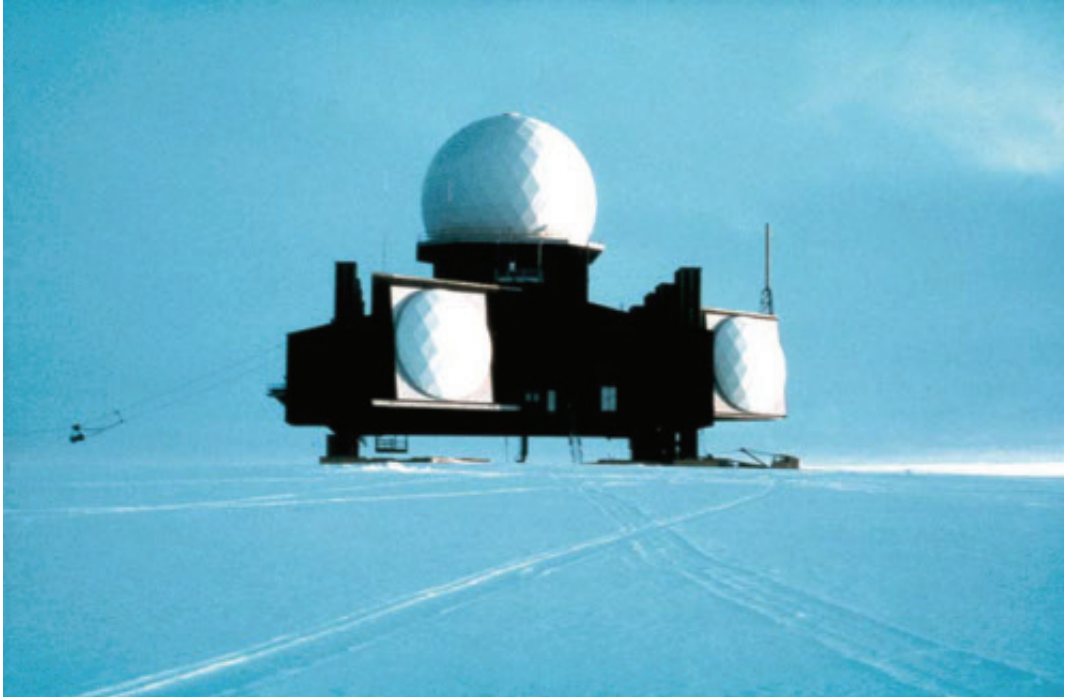
Fig. 7.2 The American radar station Dye 3 in South Greenland
