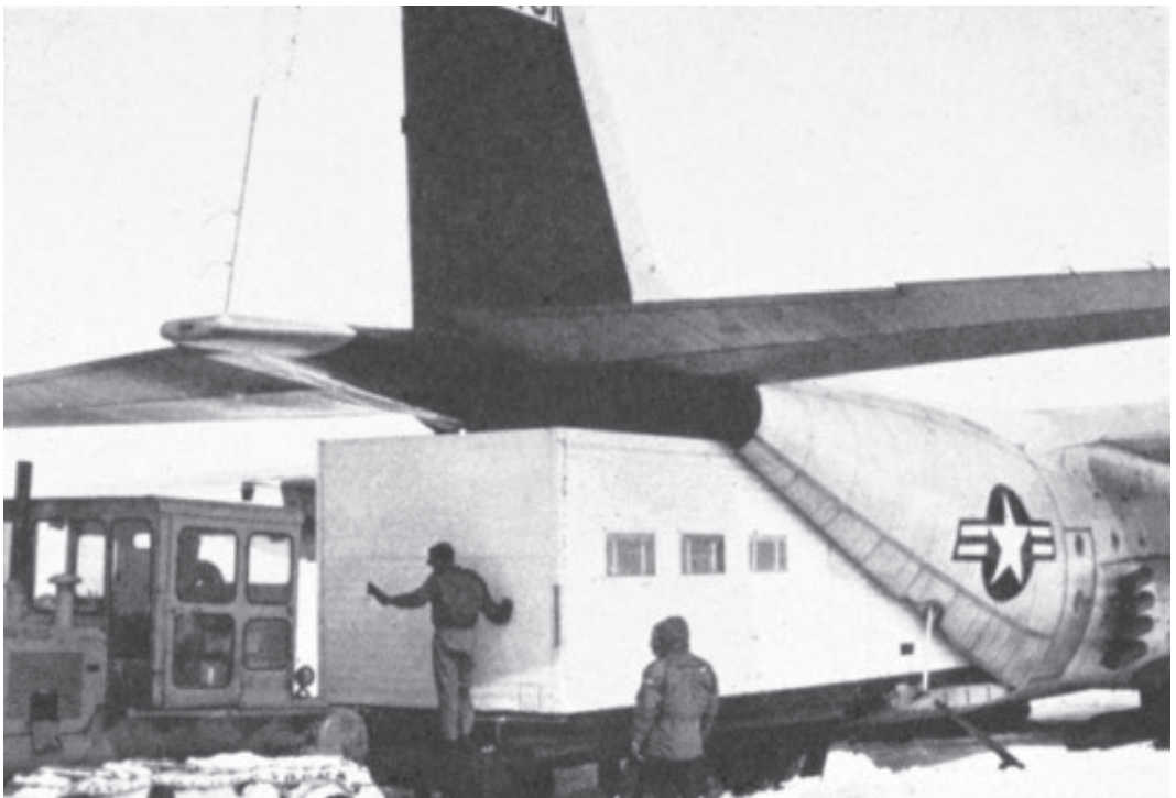
Fig. 7.1 When building the Dye stations, DAC used prefabricated houses designed to fit precisely into the Hercules aircraft. The houses were fully equipped with sleeping quarters, kitchen and bathroom. They were usable a few minutes after unloading upon the snow. Photo: DAC.
