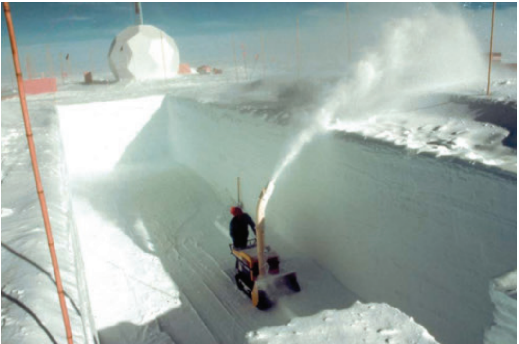
Fig. 12.3 Excavating the drill hall at Summit
